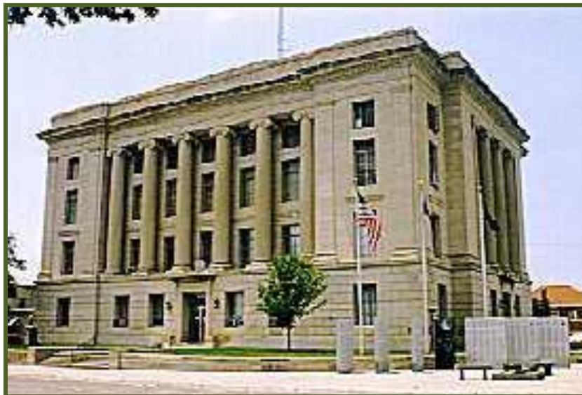
Figure 4 Rooks Co. Courthouse-Stockton, KS
